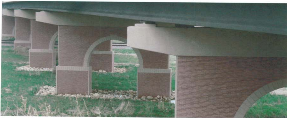
Precast thin brick panels eliminate the need for lintels, sills, weep holes and tie rods.
